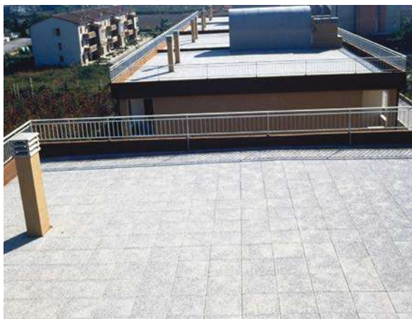
Tetto piano pedonabile
